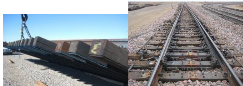
#20 Turnout With Under-tie Pads
